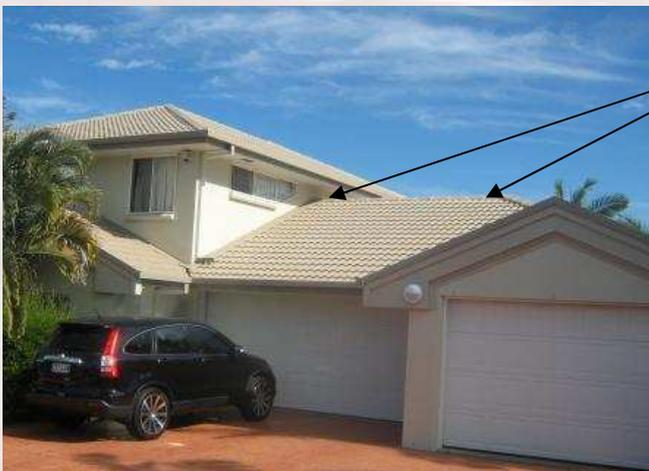
3. Condition of ridge capping. E.g. condition of bedding and pointing. Major or minor cracks in the bedding and pointing can cause leaks or dislodgement of the ridge.
