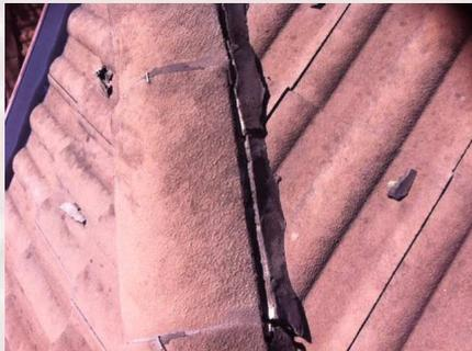
2. Check for broken ridge and gable tiles, which may cause leaks
