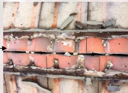
6. Condition of valley irons. E.g. do they need replacing due to rust?
