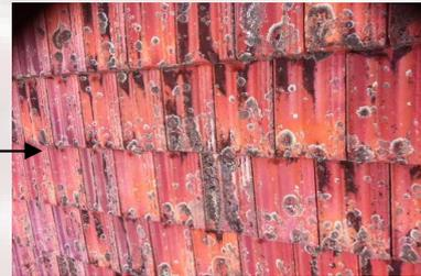
9. Fixing methods: e.g. have the tiles been secured down properly? During high wind, if tiles are not secured properly they may lift, causing the loss of parts, or in extreme cases, all of your roof.
